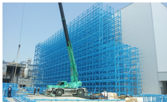
Rack Supported Building(RSB) 설치
